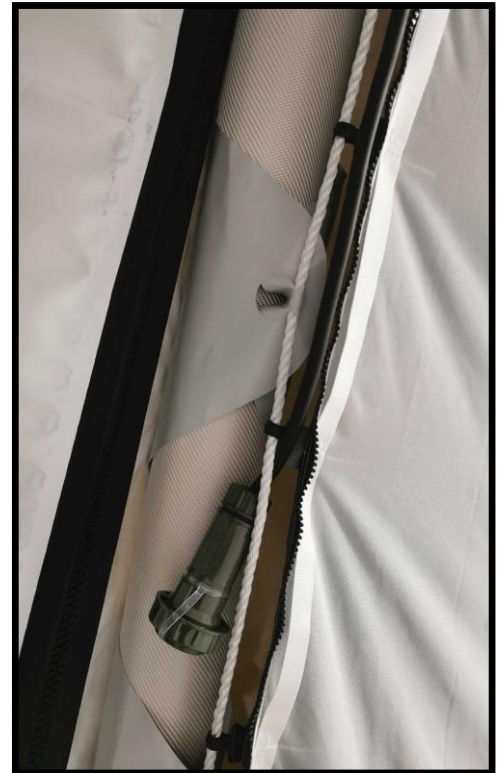
Figure 30. Inner Liner hooks' attachment to the rope along the air beam.
