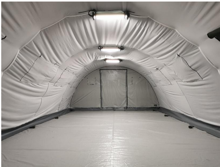
Figure 31. Installed inner liner with light and power distribution system.
