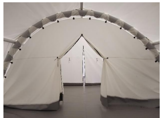
Figure 32. Partition wall installed directly on the air beam.
